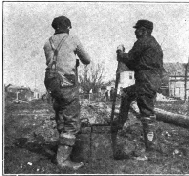
Fig. 12.—View Showing Method of Using Iron Barrel in Digging Pole Holes in Soft Ground.
